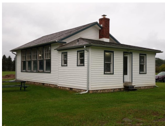
Hicks School after the move
